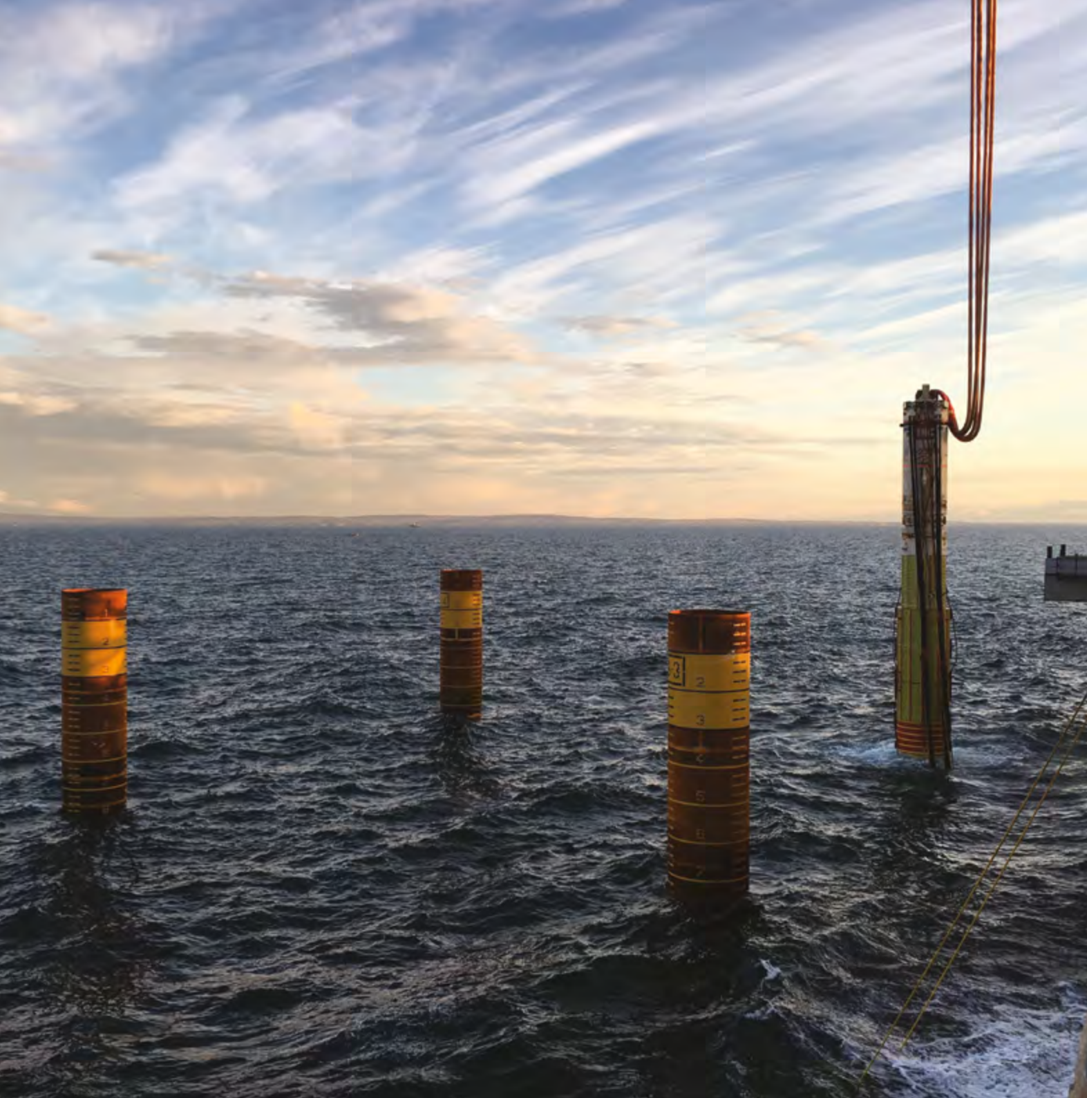
Above: PIF being lowered in to the water.
