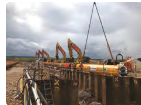
Above: Direct Pipe Thruster at the Portgordon export cable landfall site
