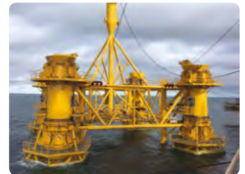
Above: PIF being lowered in to the water.
