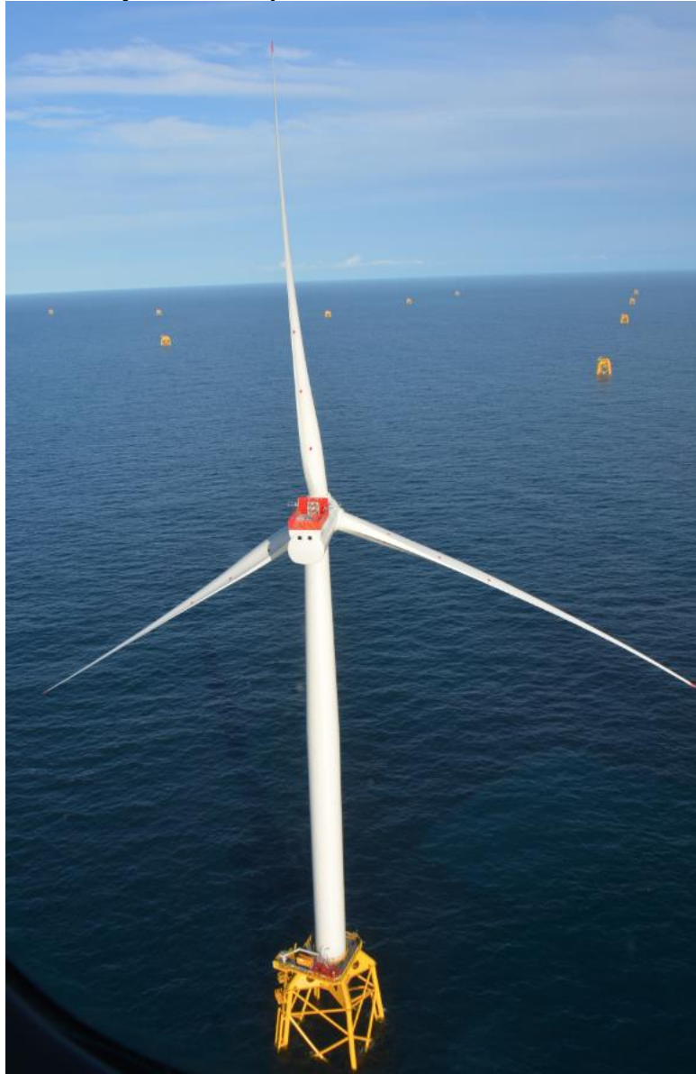
Fig. 5 Siemens SWT-7.0-154 WTG installed at Beatrice OWF
