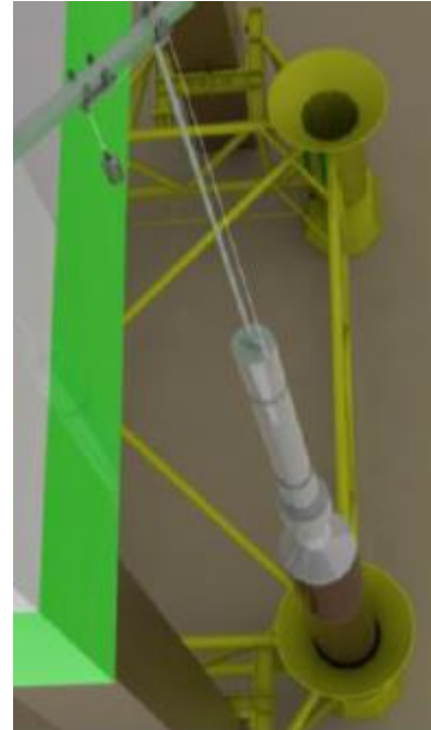
Figure 10 Hammer positioned on pile
