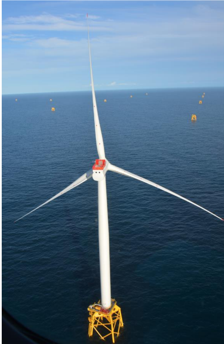
Fig. 4 Siemens SWT-7.0-154 WTG installed at Beatrice OWF
