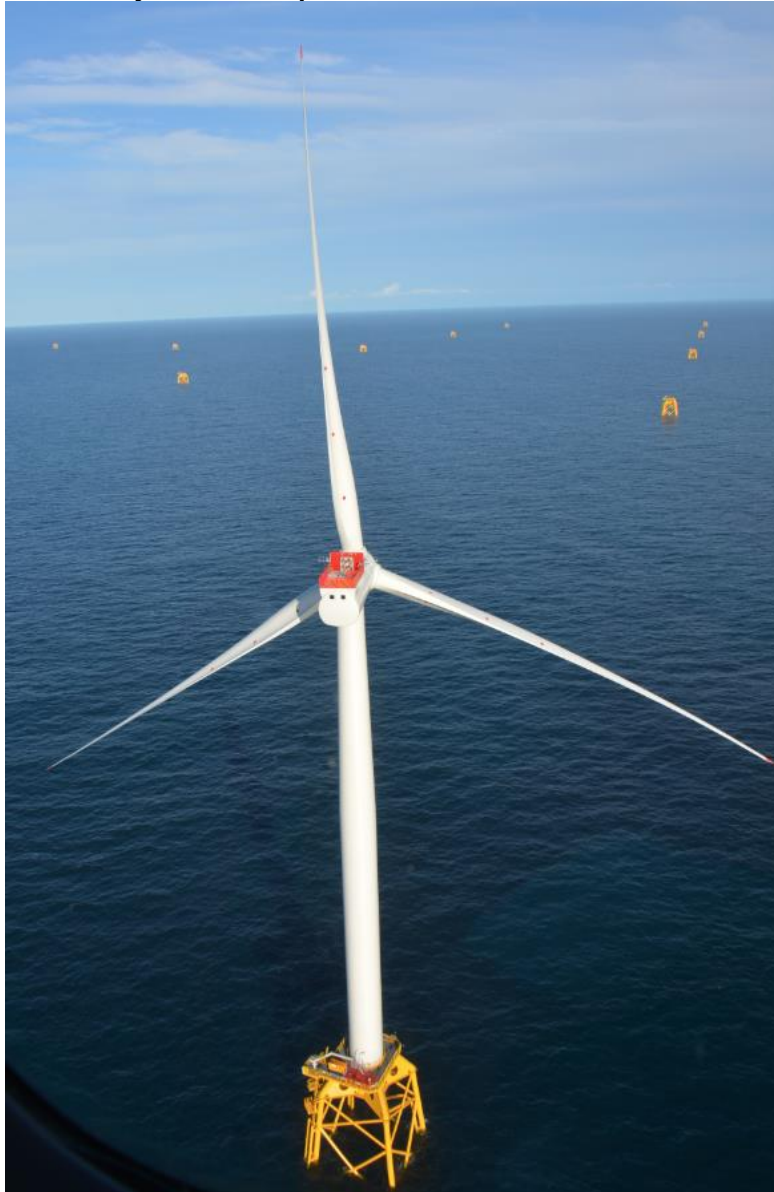
Fig. 5 Siemens SWT-7.0-154 WTG installed at Beatrice OWF
